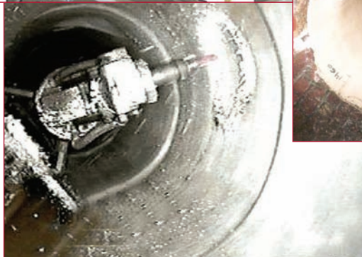
Robots re-establish the service connections.
