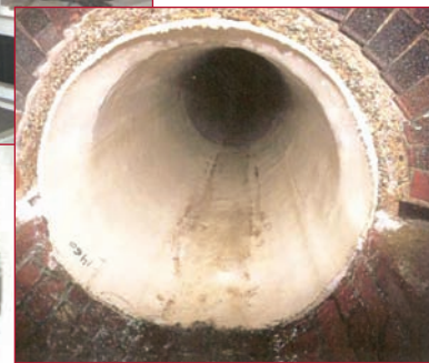
The rehabilitated pipe.
