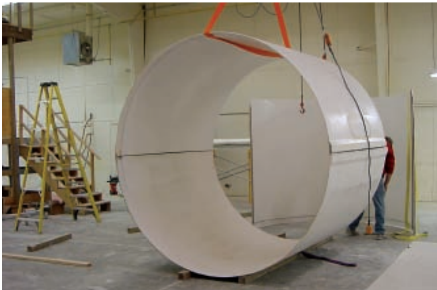
ArmorGRIP® panels by Insituform are assembled to rehabilitate a large sewer line.
