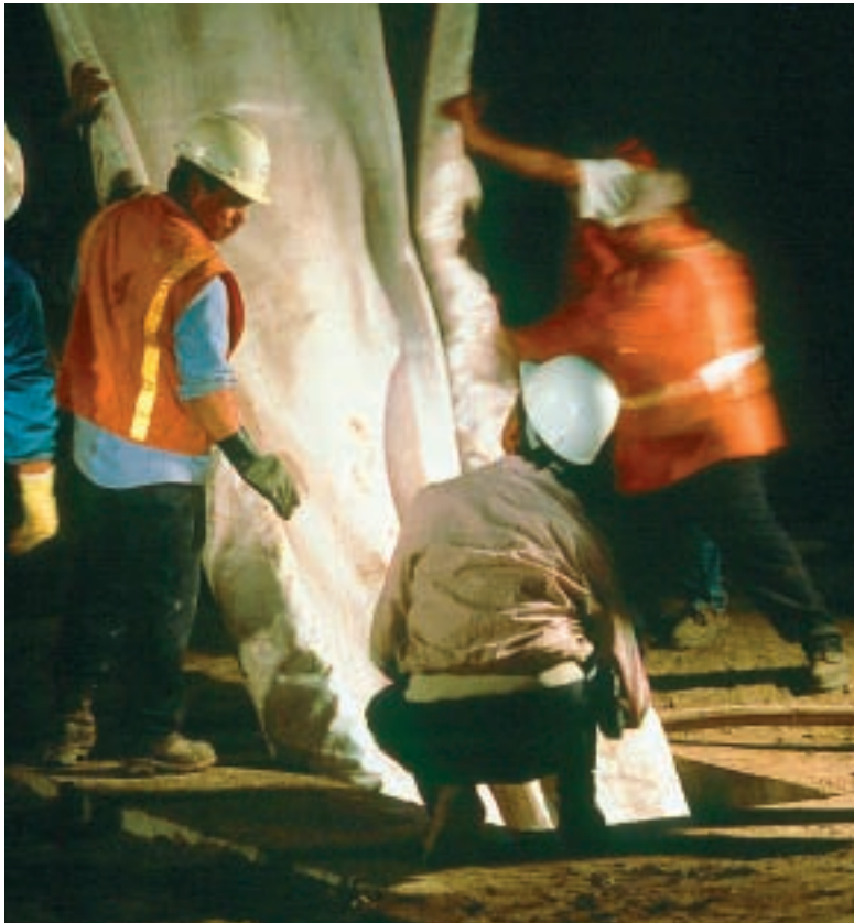
Cured-in-place pipe installation.
